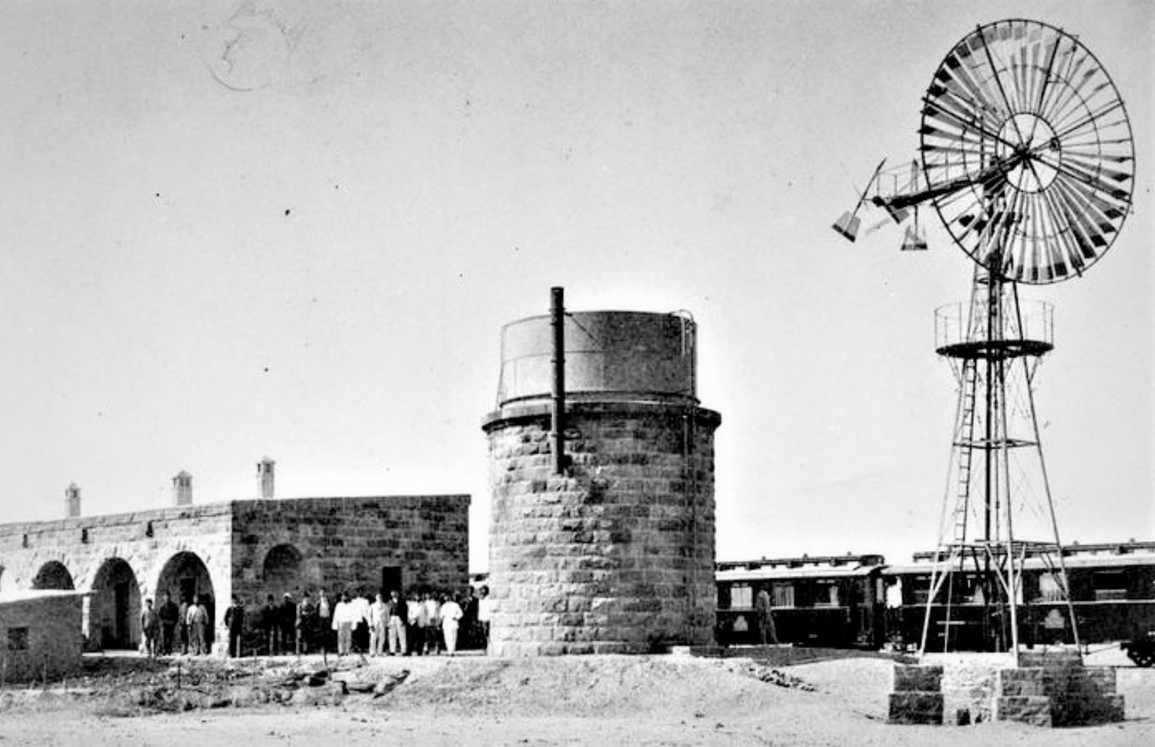
Hejaz Railway station at Dhat al-Hajj, 1916 – Author, J. H. Halladjian, Imperial War Museum, public domain, Wikimedia. Windmills pumped water from wells to above ground water tanks.
