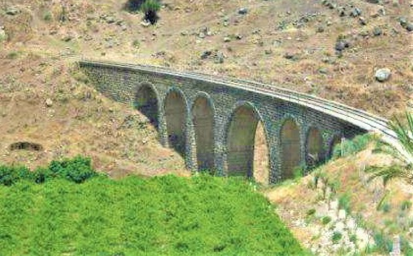
Hejaz Railway masonry viaduct– esyria.sy/sites
