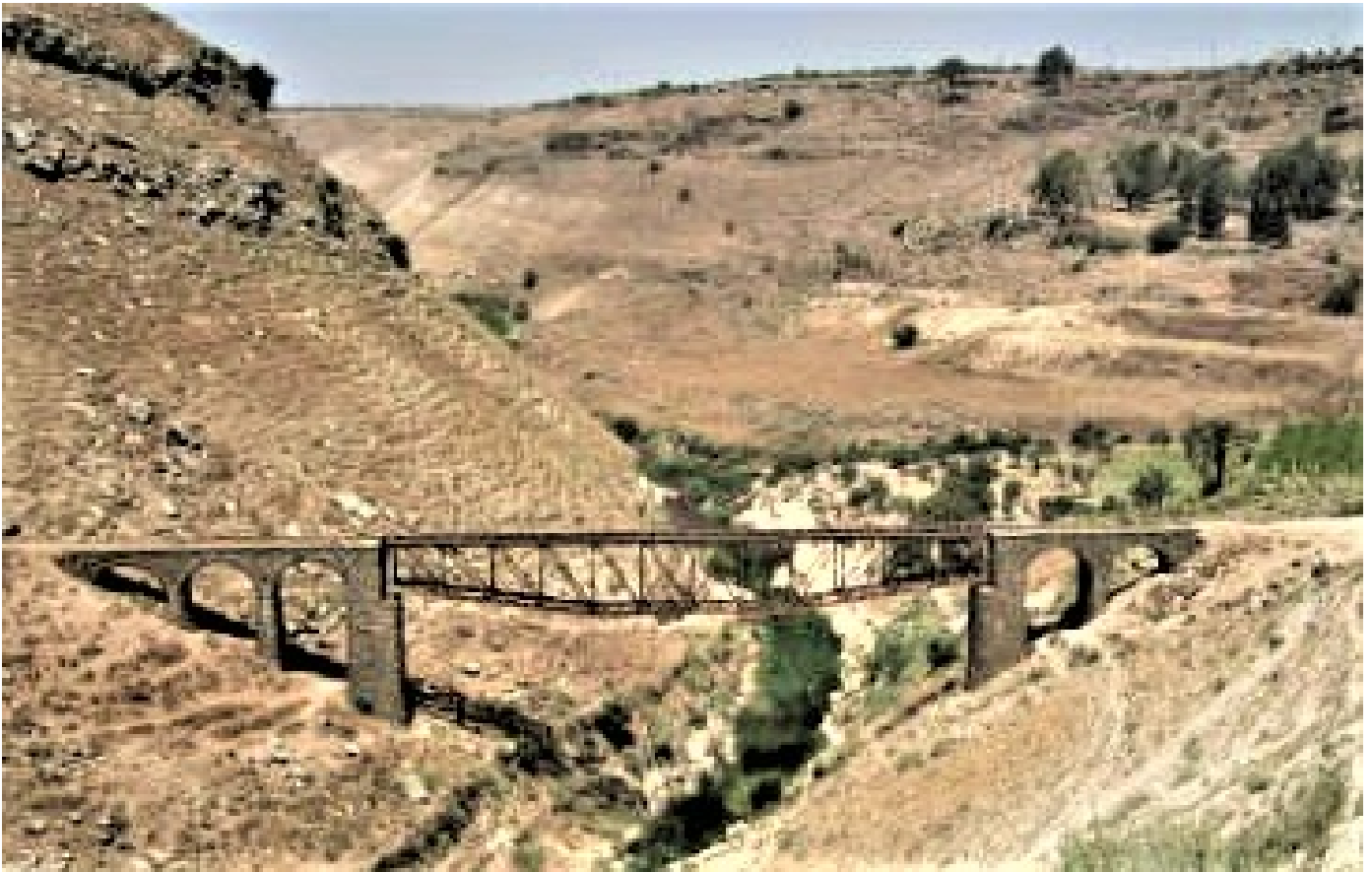
Tell el Shehab Bridge in Yarmouk Valley – esyria.sy/sites
